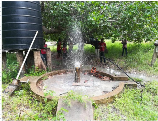
Flushing of 1st well in Mavunja refurbished
