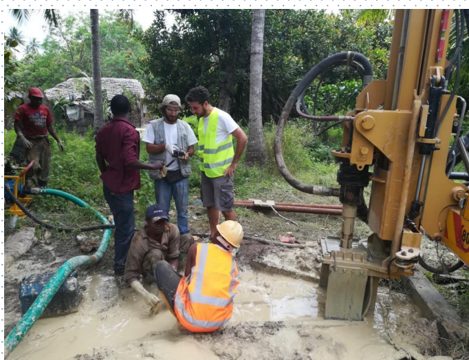
Excavation of the new Mavunja well.
